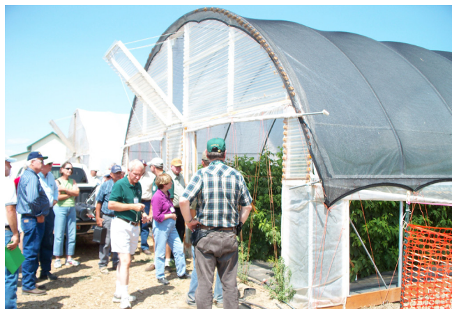
Figure 3: Woven shade cloth fabric installed on the exterior of the high tunnel. (Photo by Steve Hawkins)
