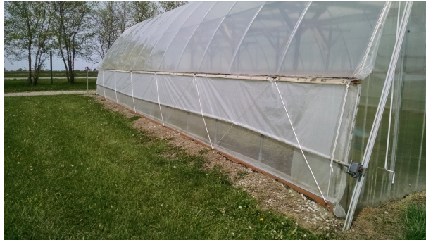
Figure 2. Insect screens installed on a high tunnel.
