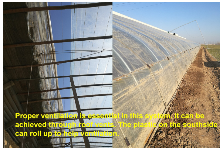
Figure 3. Passive solar greenhouse ventilation (Photo by Wenjing Guan).
