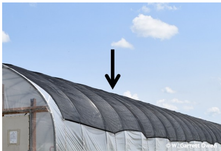
Figure 15. Exterior shade cloth utilized to limit solar ambient light into the greenhouse environment, thereby reducing daily light integral. Photo by: W. Garrett Owen, OSU.
